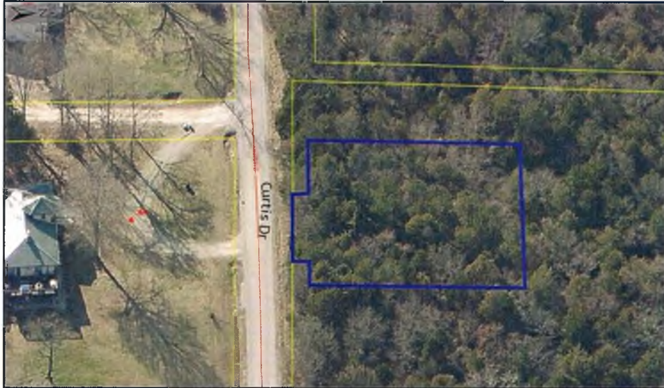
MO-15 Powersite Telecommunications Tower 300 Block Curtis Drive, Forsyth, MO Division III Permit Case # 2016-0028 Pictometry – View from the East
