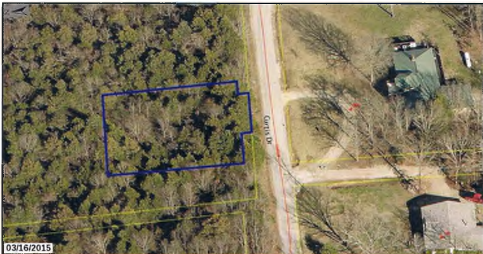
MO-15 Powersite Telecommunications Tower 300 Block Curtis Drive, Forsyth, MO Division III Permit Case # 2016-0028 Pictometry – View from the West
