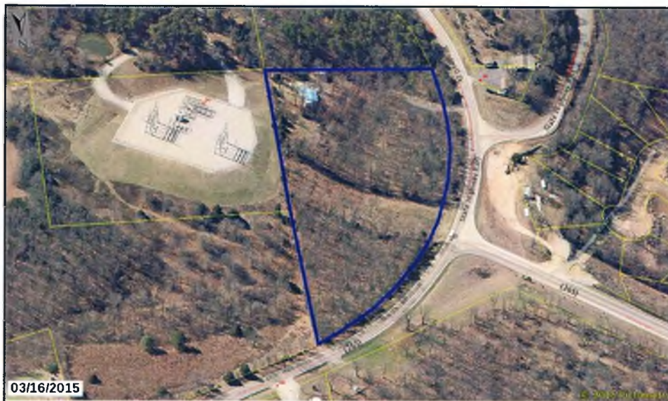
Windmill Road Telecommunications Tower 169 Windmill Road, Hollister, MO Division III Permit Case # 2016-0024 Pictometry – View from the North
