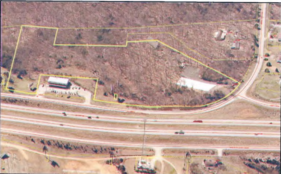
Stonegate Glass Chapel 11027 State Highway 176, Walnut Shade, MO Pictometry – View from the East
