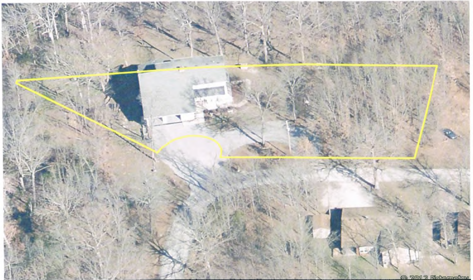
410 Newton Road Nightly Rental 410 Newton Road, Ridgedale, MO Division III Permit 2015-0014 Pictometry – South View
