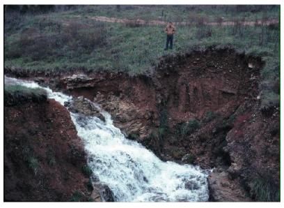
Figure 3-11: Erosion at Silver Creek Dam
