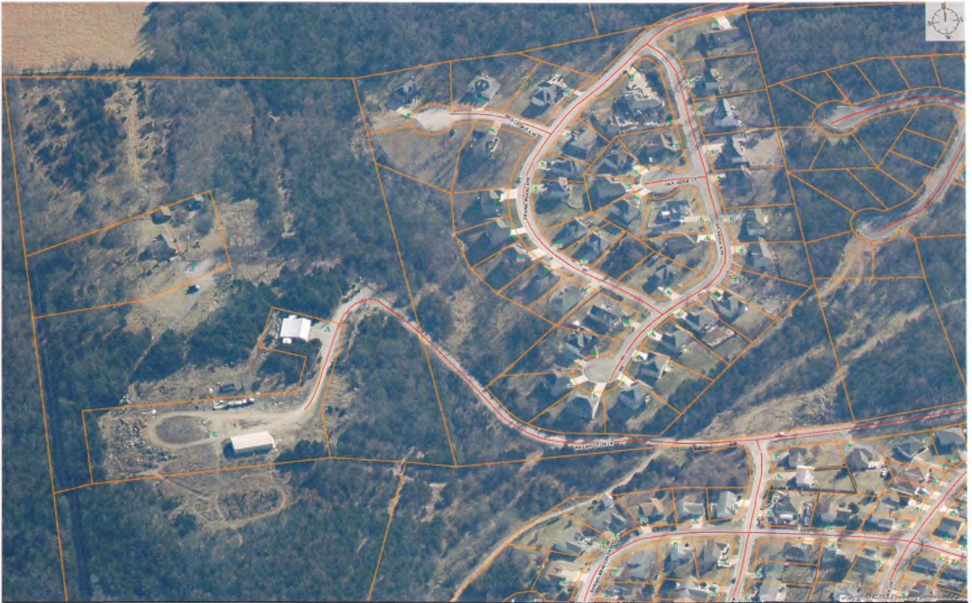
Walkington Affordable Housing Division III Special-Use Permit 2014-0003 Pictometry – View from the West
