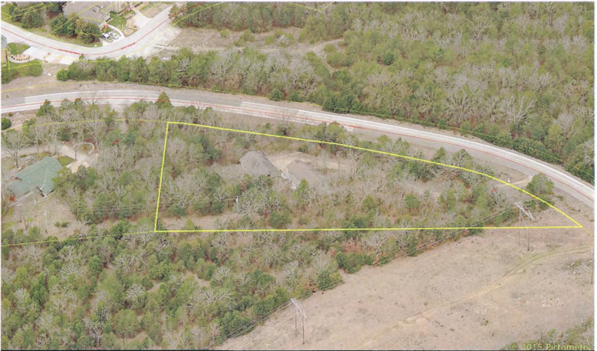
615 State Highway P Nightly Rental 615 State Highway P, Hollister, MO Division III Permit Case # 2015-0024 Pictometry – View from the East
