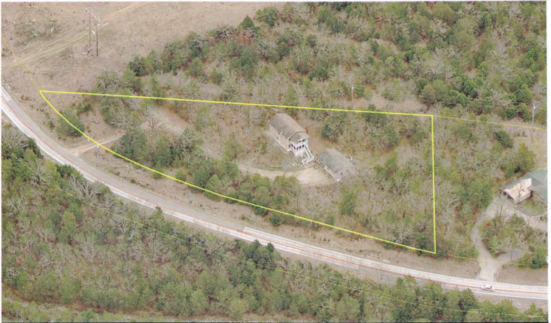
615 State Highway P Nightly Rental 615 State Highway P, Hollister, MO Division III Permit Case # 2015-0024 Pictometry – View from the West
